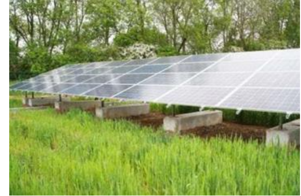
Panels with Concrete Feet
